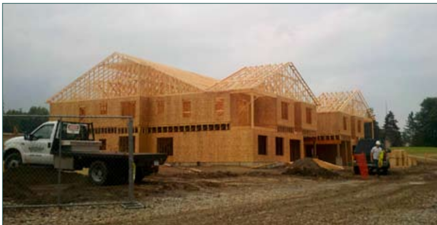
New Broad Street Apartments are under construction.
