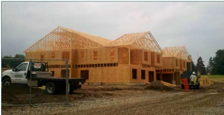
New Broad Street Apartments are under construction.
