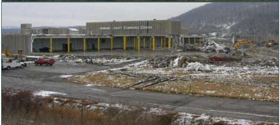
Former A&P Plant makes way for new shopping plaza.
