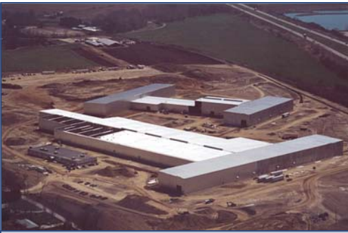
As the first Empire Zone Project in the State of NY, Vulcraft set the tone for STEG to develop additional shovel ready sites throughout the community. This paid off in February of 2009 when CVS announced the development of a 751,000 sq ft distribution center in the Town of Chemung, creating 600 new jobs.
