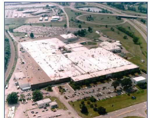
In 2006, STEG assisted with the retention of Eaton and over 200 jobs in the former Westinghouse building which helped leverage the sale of the building from Viacom to a private development firm.
