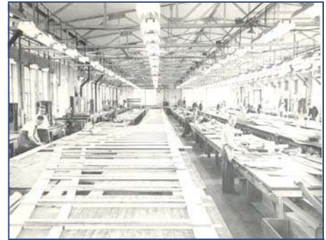
The former American Bridge Plant in Elmira Heights has been transformed into a rail car manufacturing facility and served as a base of operations for a number of companies in this industry through the 90's until CAF USA purchased the facility in 2001 making it their North American headquarters.
