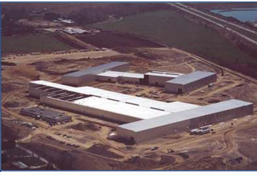
As the first Empire Zone Project in the State of NY, Vulcraft set the tone for STEG to develop additional shovel ready sites throughout the community. This paid off in February of 2009 when CVS announced the development of a 751,000 sq ft distribution center in the Town of Chemung, creating 600 new jobs.
