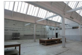
Aging Building Stock
